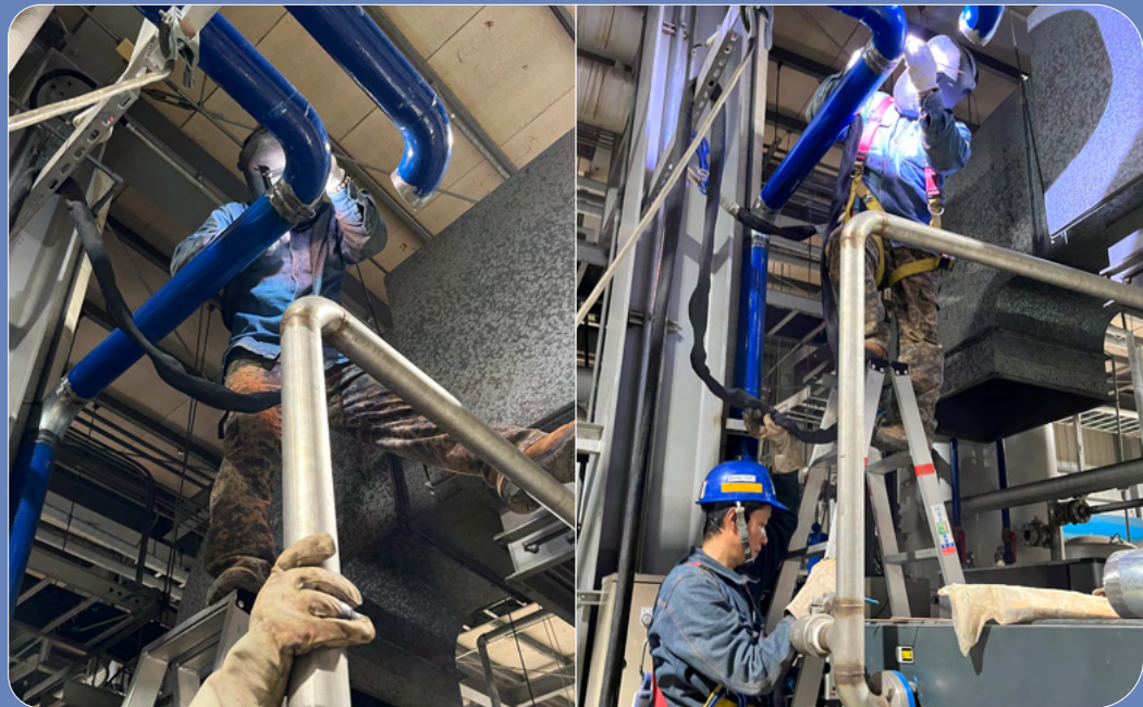
▲ When the contractor stepped on a pipe during work, the supervisor immediately stopped it and asked for improvements. Work can only continue after ensuring that safety measures have been implemented.
