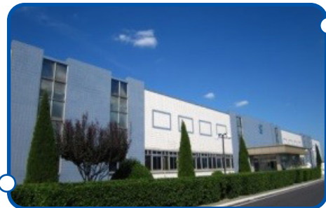
Shandong Site Yangxin Everwell (assembly and testing site)
